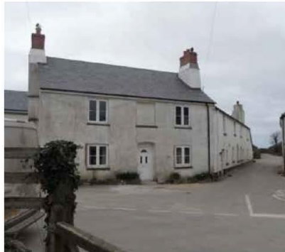
3. Existing building types. Note expressed chimney character
